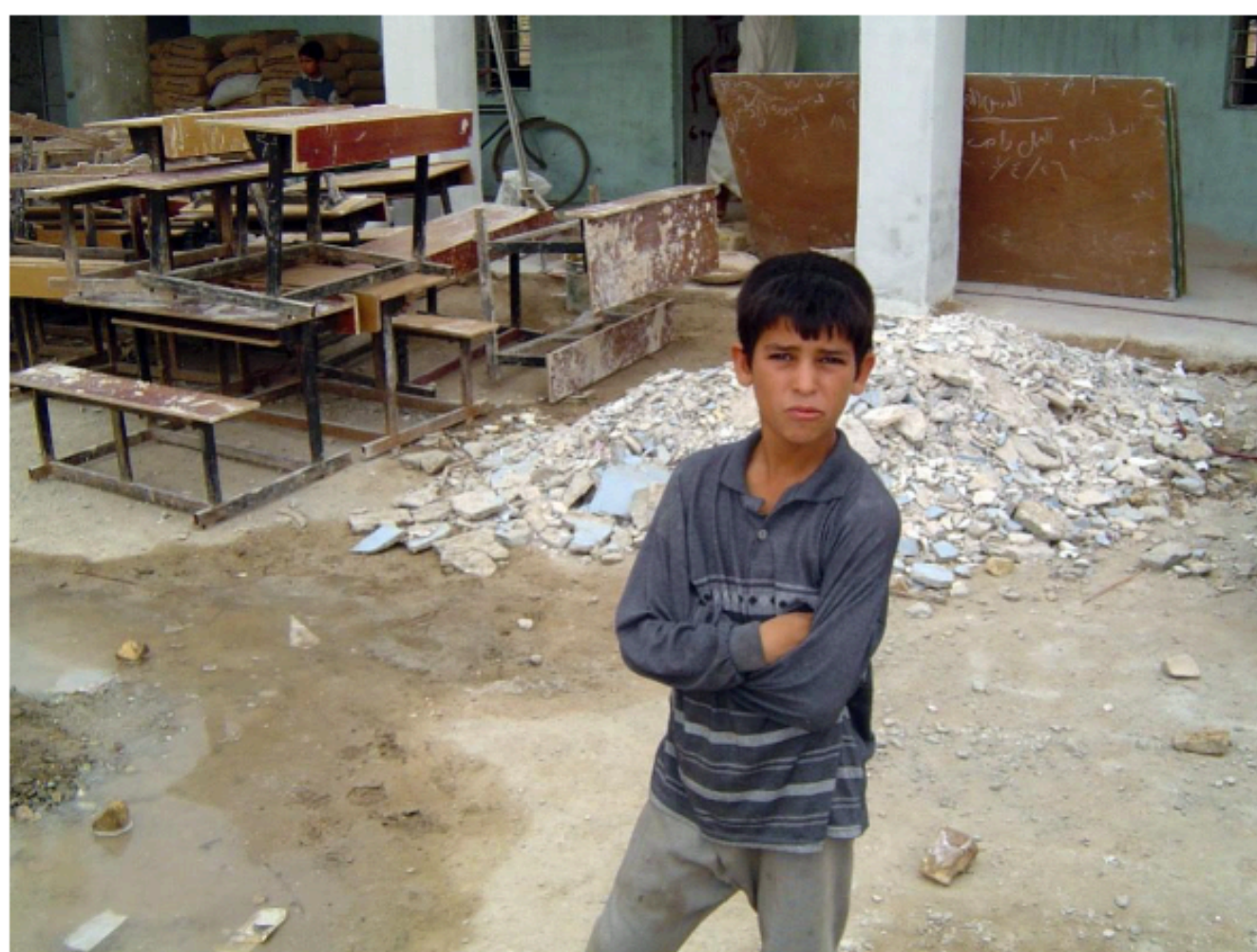
Bahkan School Project before construction.
